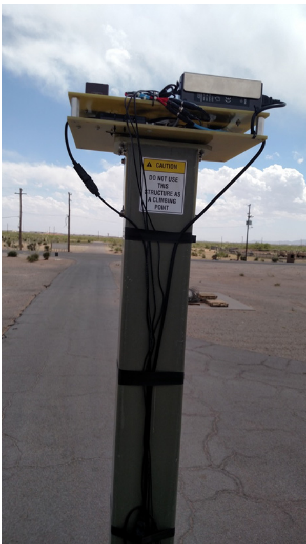
Figure 13: 4.5-Ft riser placement.
